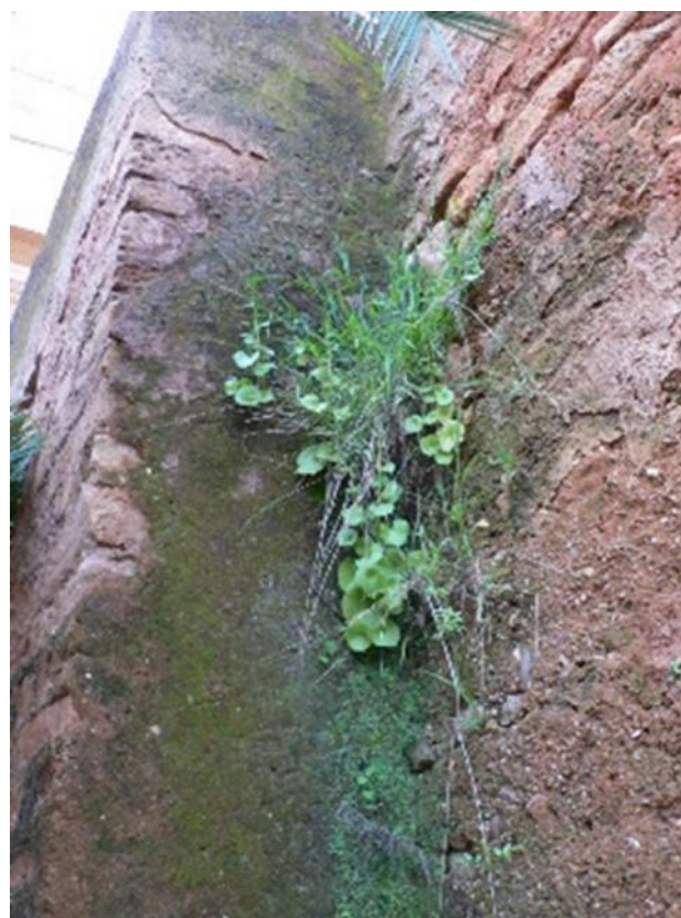
Fig.8: Terracotta brick wall of the gate covered with bryophytes that maintain a high degree of moisture on the masonry
