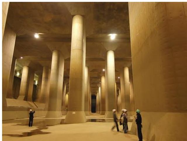
Fig. 7. "Water pressure control bath" (size 178x77x18 meters)
