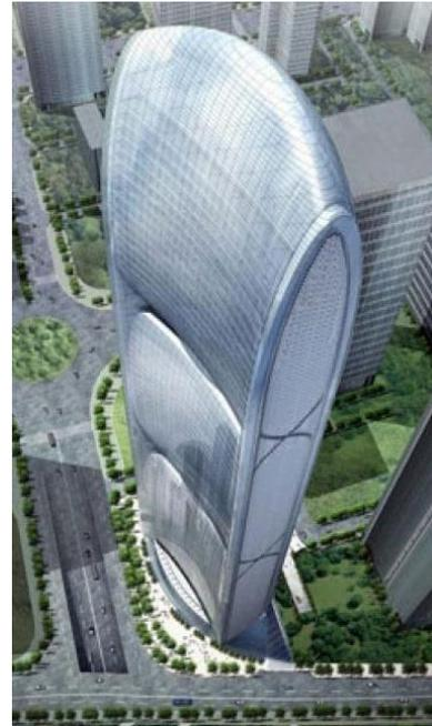
Fig. 14. Zero-energy skyscraper «Pearl River Tower» [23] (spiral "wind vents" are visible on the right side of the house, solar panels are on the facade)
