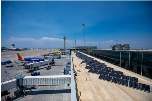
Fig.1: Photovoltaic PV Solar System at Denver International Airport
